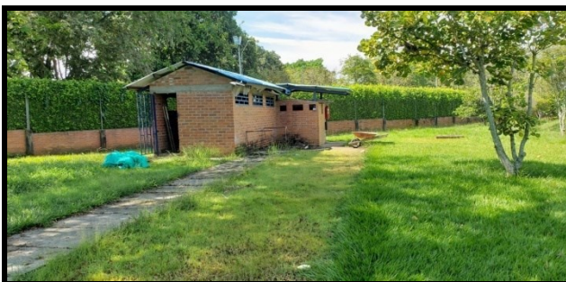
Foto 1. PTAR COLEGIO BRITANICO THE BRITISH SCHOOL LTDA.
